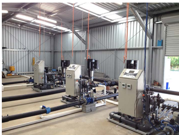
Netajet control and fertiliser injector system for berries – a solenoid-controlled venturi injection system. Image by John Witherspoon.
