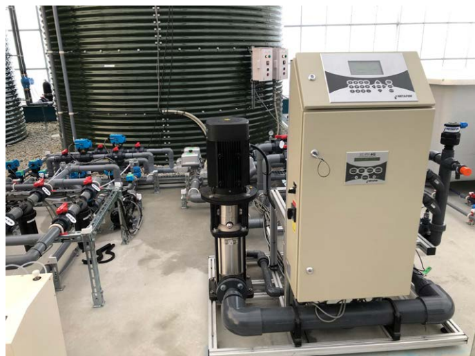
Netajet machine: The venturi requires a pressure differential to operate. The pressure differential is created on the machine, not the mainline. Image supplied by Netafim.
