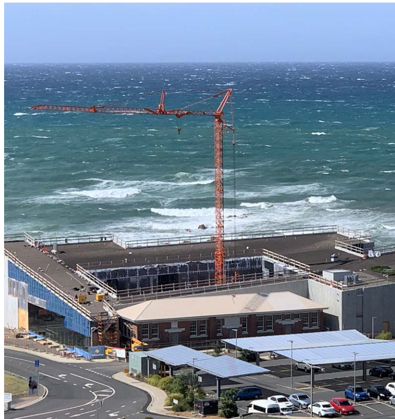
The university campus's green roof under construction. Image supplied by Fytogreen.
